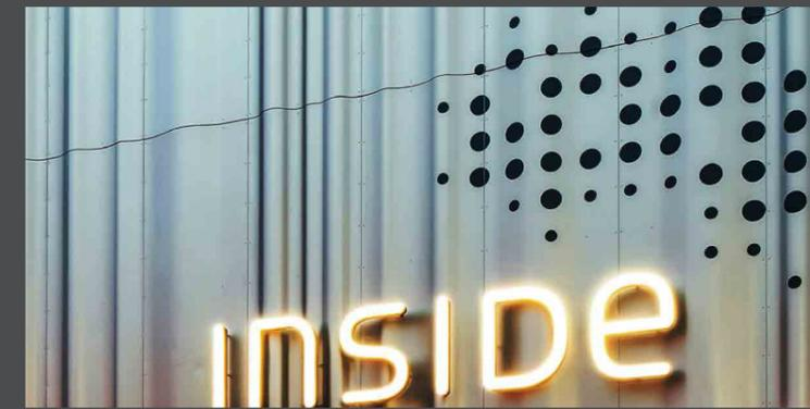
Like a golden curtain, the ALUCOBOND® elements ripple across the building. The round recesses above the lettering are backlit and make the curtain glisten.
