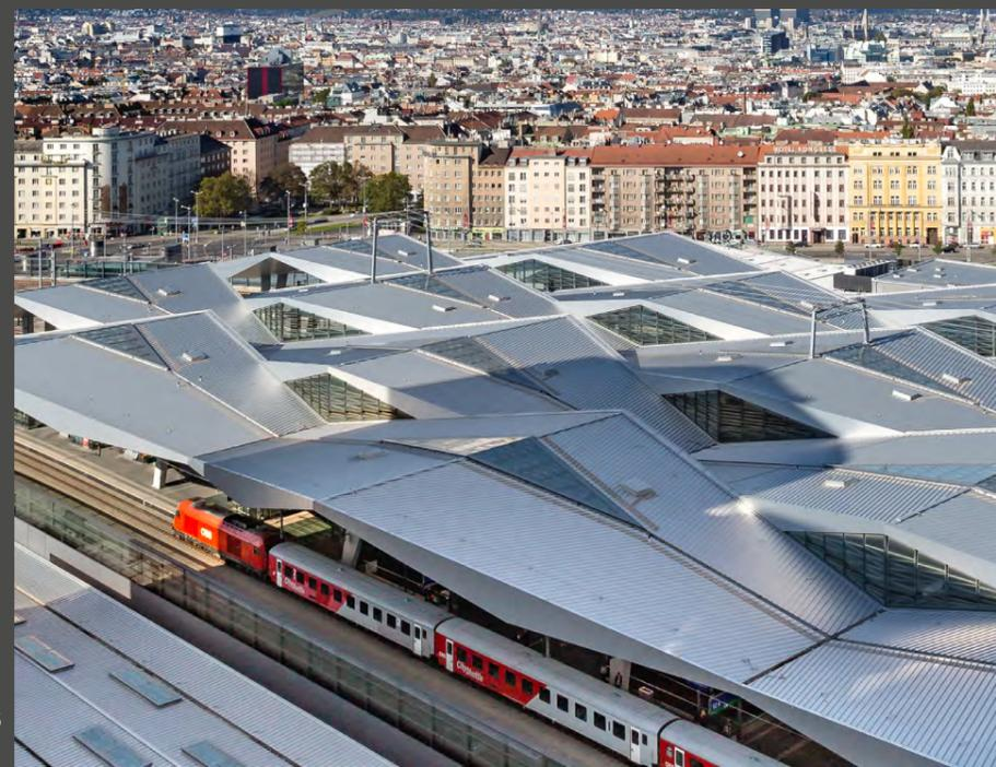
Visually there are ten; structurally five roof bands. Undulating above the rails towards the east, they converge and diverge to form rhomboid shapes at specific points.
