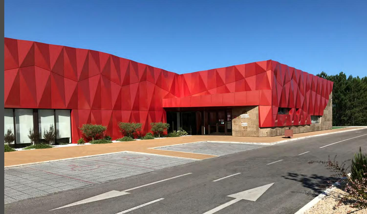
Like the earth consisting of fire and stone, at least figuratively. In reality, the polygonal landscape is made of ALUCOBOND<sup>®</sup>.
